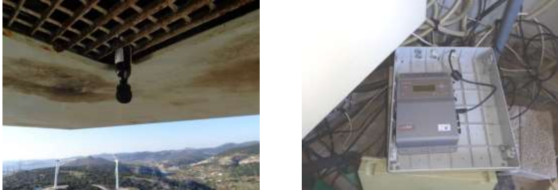
Figure 7. Installation of a bat detector system at NEG MICON/750 kW wind turbine at CRES demonstration wind farm
